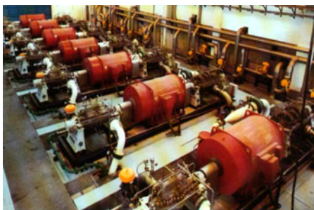
Fig. 2. Original plant layout with Francis ERT's and first retrofit to Pelton type ERT's.
