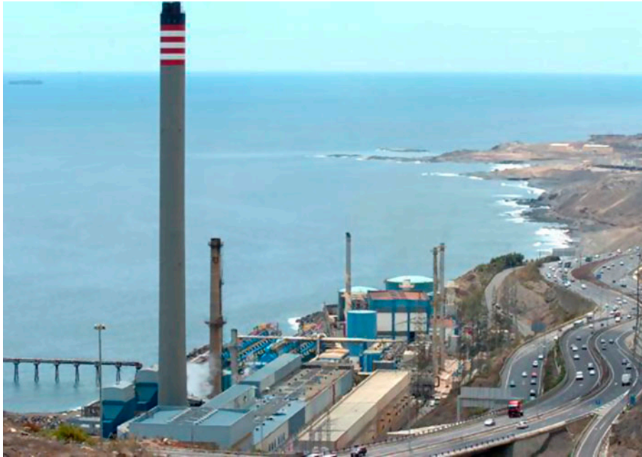
Fig. 1. Las Palmas III SWRO plant location.
