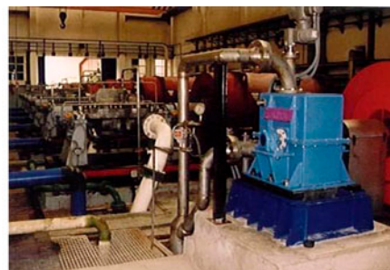
Fig. 2. Original plant layout with Francis ERT's and first retrofit to Pelton type ERT's.
