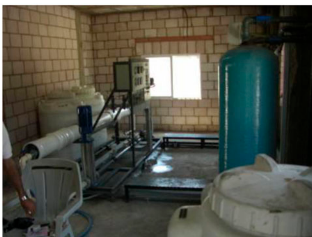
Fig. 7. View of a 20 m 3 /d RO unit, Jordan Valley. Source: NERC.
