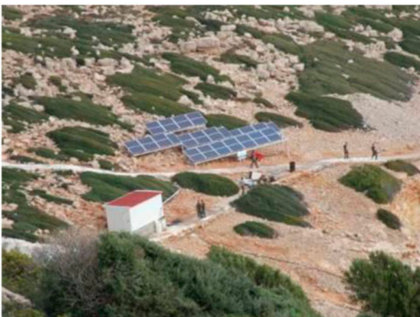
Fig. 4. 20 kWp PV unit, Strogili island, Greece.
