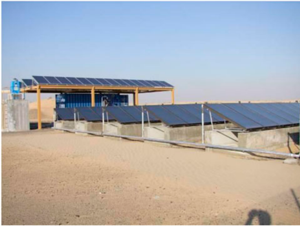
Fig. 20. View of a solar thermal powered MEH system installed in Dubai (UAE). Plant capacity 5,000 l/d and 170 m 2 solar thermal collectors [25].
