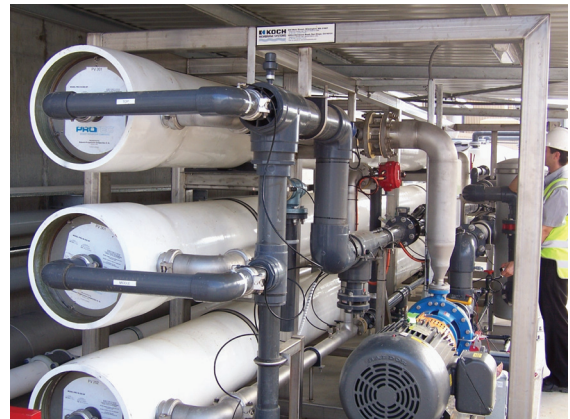
Fig. 4. MegaMagnum ® reverse osmosis system at Joe White Maltings in Australia.
