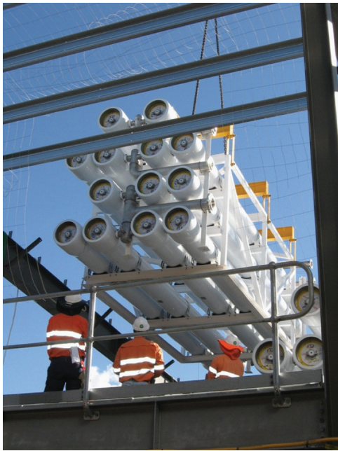
Fig. 6. Installation of RO rack at Bundamba AWTP.
