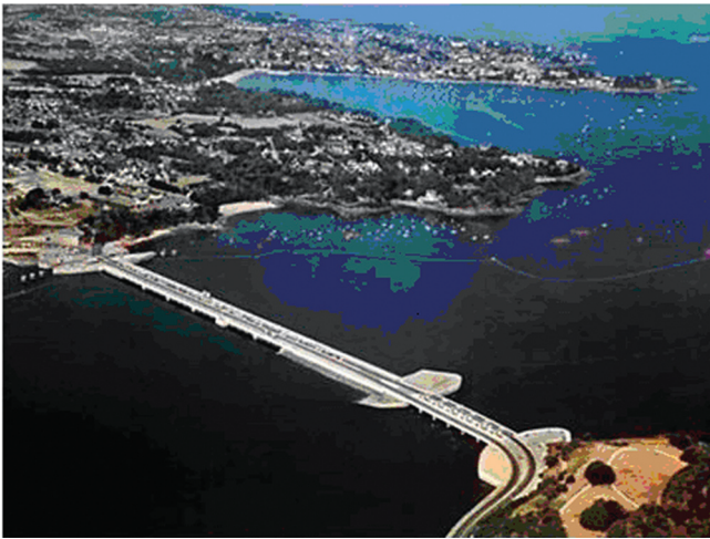
Fig. 21. The tidal power station at the mouth of the Rance River at Saint Malo (Bretagne). The 750 m long dam separates the storage reservoir from the open sea.
