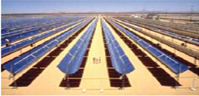
Fig. 18. This picture of a linear parabolic solar power station in California visualizes the extreme floor space required by solar power plants.
