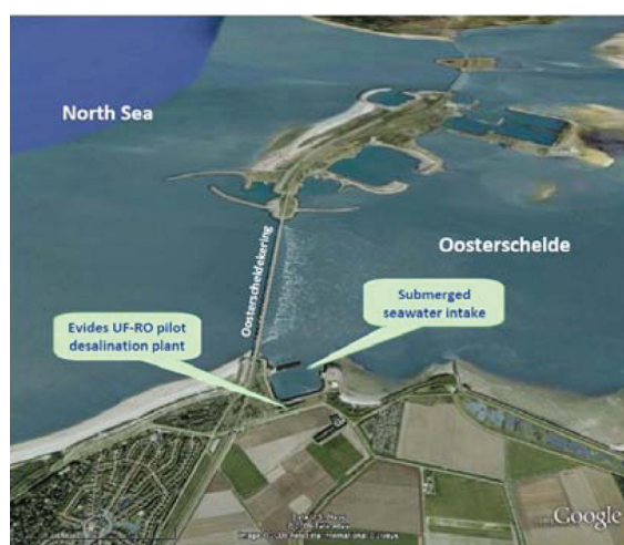
Fig. 2. Location of the UF-RO plant and its raw water intake (satellite image from Google Earth).
