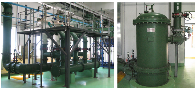
Fig. 7. Disc filter and cartridge filter.
