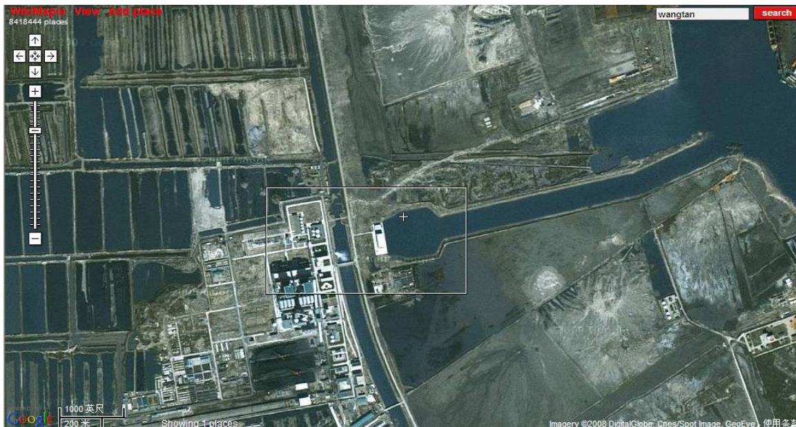
Fig. 3. Satellite picture of intake channel and pond.
