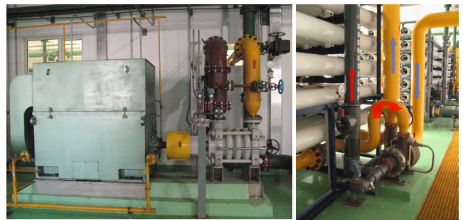
Fig. 8. Feed pump and turbocharger.
