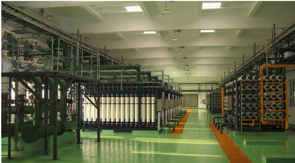
Fig. 9. UF (left) and SWRO trains (right).
