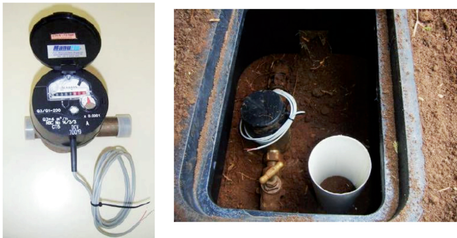
Fig. 1. CT5-S Meters (left) and installed (right).
