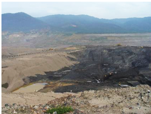
Fig. 2. High-volume strip mine ČSA with retention reservoir for mine waters transfer pump station.
