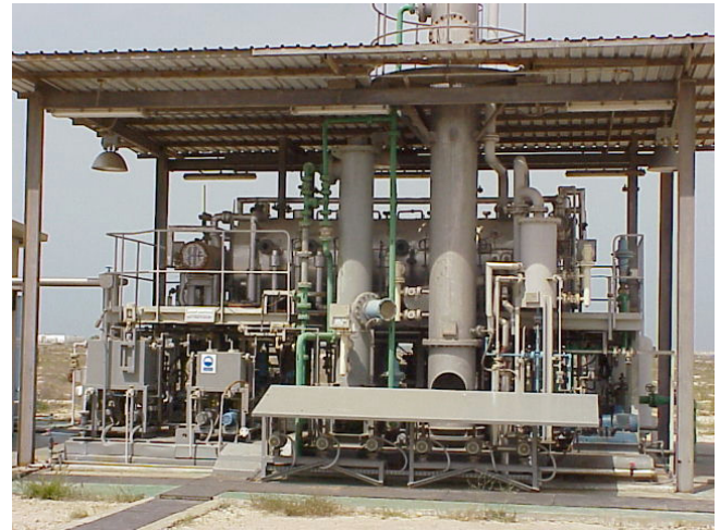
Fig. 2. MSF pilot plant, capacity 20 m 3 /d.
