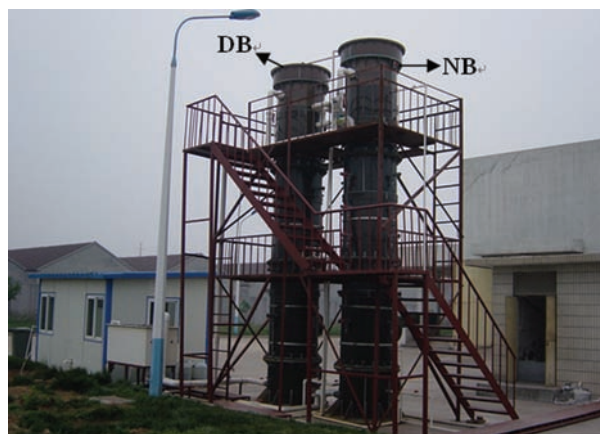
Fig. 2. On site photograph of the pilot-scale experimental apparatus.
