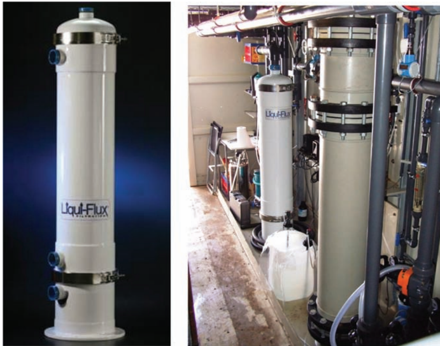
Fig. 3. Sand filter and ultrafiltration source: MEMBRANA/WAT module in the container [4,5].
