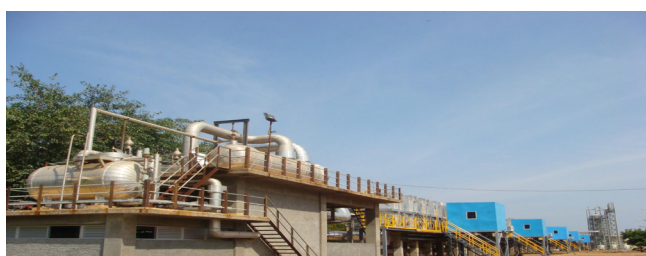
Fig. 3. Desalination plant at nuclear power station Kalpakkam, India.
