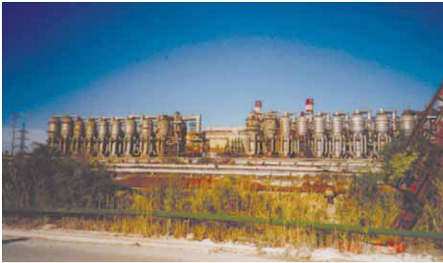
Fig. 1. Distillation units at Aktau, Kazakhstan.
