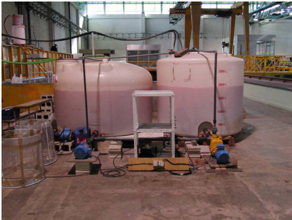
Fig. 13. The discharge storage tanks.
