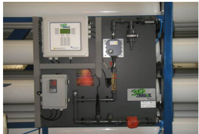
Fig. 3. Nalco Trasar 3-D device.
