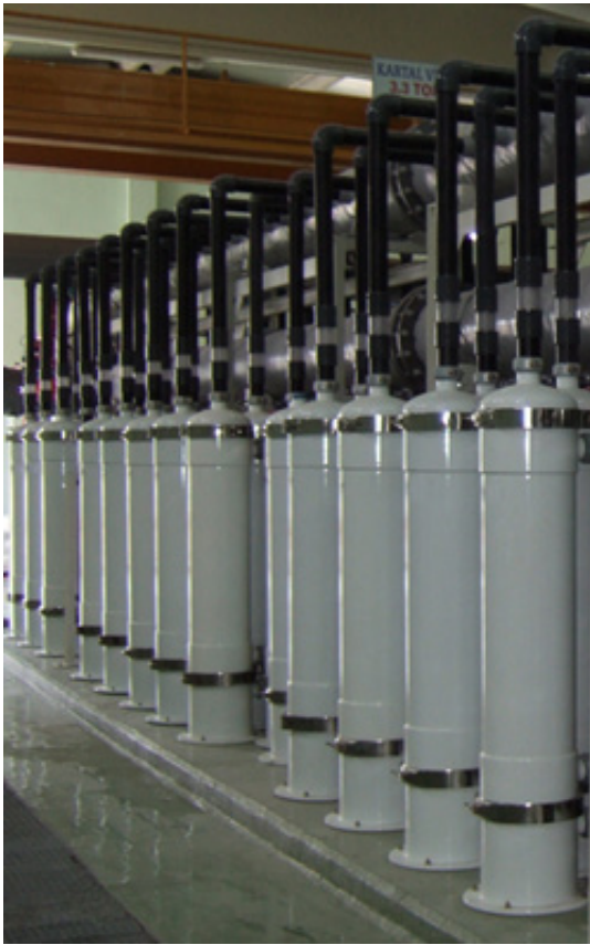
Fig. 6. Ultrafiltration rack.
