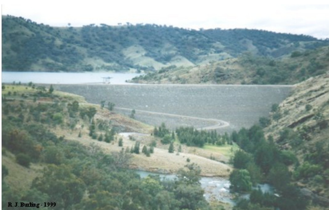
Fig. 4. The Split Rock rock fill dam in NSW is very similar in size and shape with a wall length of 469 m, a height of 66 m and a fill volume of 1.1 million m 3 .
