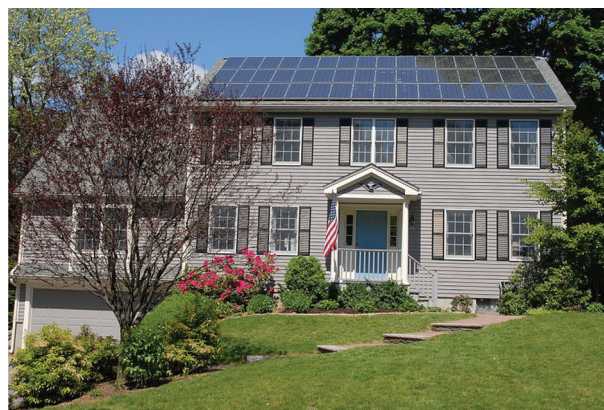
Fig. 7. PV distributed system on a house [12].
