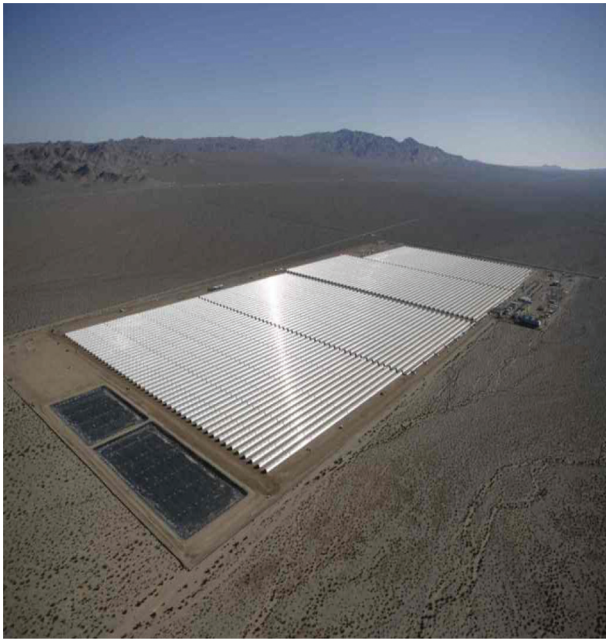
Fig. 9. Solar One Nevada, parabolic trough power plant with solar only heat input [17].
