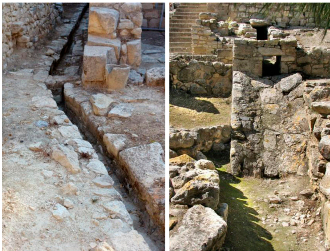
Fig. 1. Remains of central sewerage and drainage systems at Knossos “Little Palace” and Palace, respectively (A.N. Angelakis, with permission).
