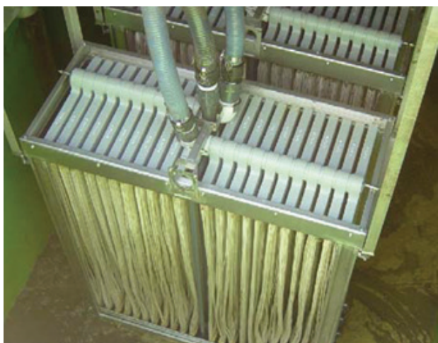
Fig. 19(b). Vacuum-driven UF system [13].
