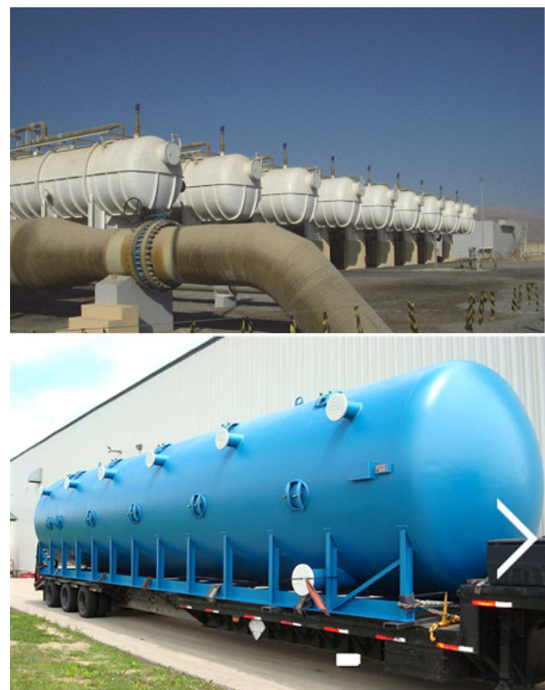
Fig. 18(b). Horizontal pressure granular media filters [13].
