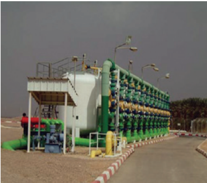
Fig. 18(a). Vertical pressure granular media filters [13].
