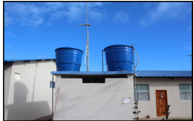
Fig. 3. Picture of typical elevated tanks in Puerto Ayora.
