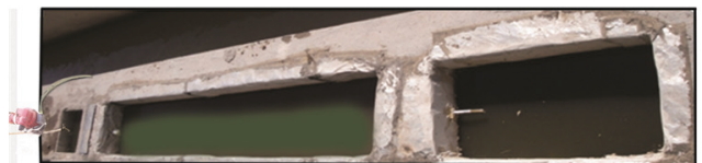
Fig. 1. View of the pilot stabilization ponds.
