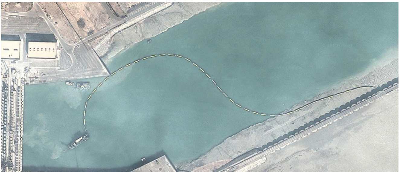
Fig. 2. Dredging process inside SPDP seawater intake.
