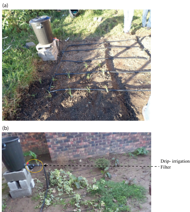
Fig. 2. Fly ash/lime filter tower connected to drip irrigation system (a) and fly ash/lime filter tower connected to a drip filter with a drip irrigation system (b).
