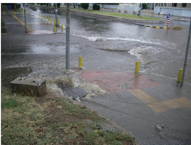
Fig. 2. Junction of Agiou Dimitriou and St. Kyriakidi Streets during a short, intense rain event.
