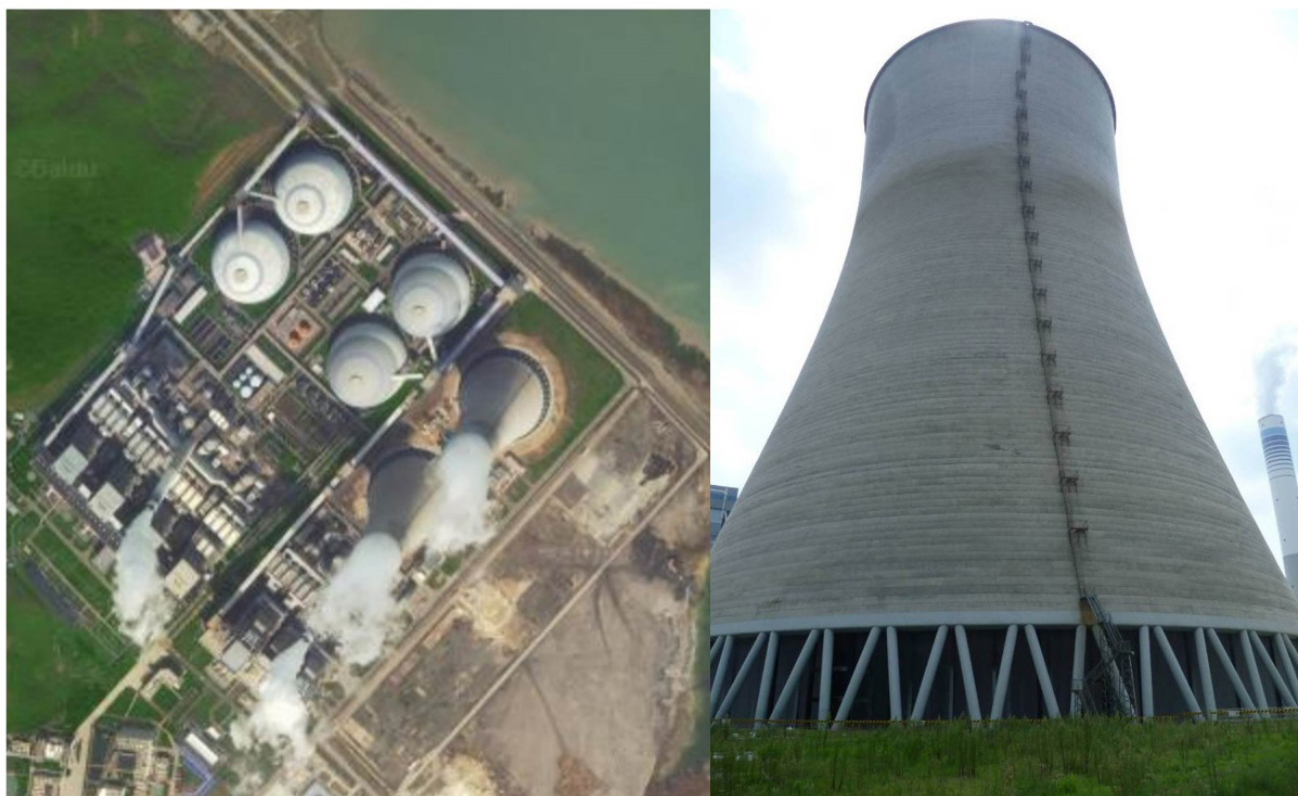
Fig. 2. Cooling tower and surroundings.
