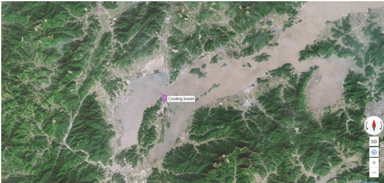
Fig. 3. Surrounding terrain of cooling tower.
