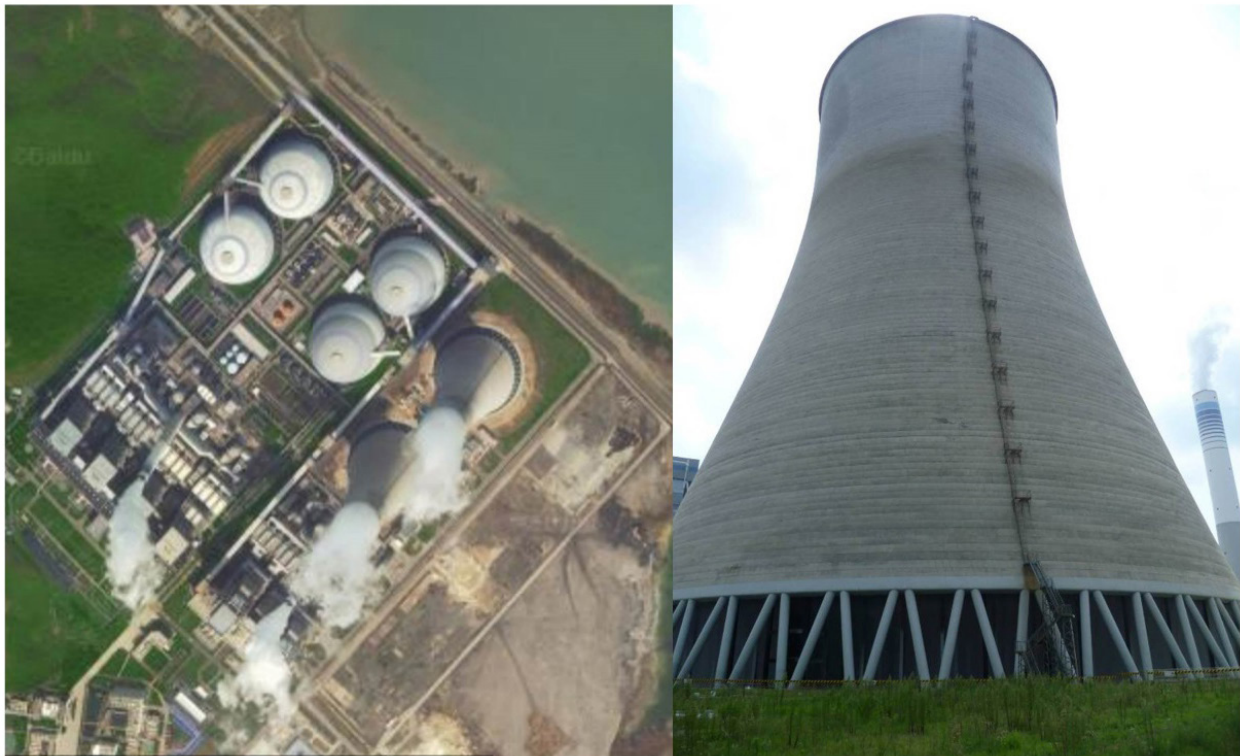
Fig. 4. Cooling tower and surroundings.
