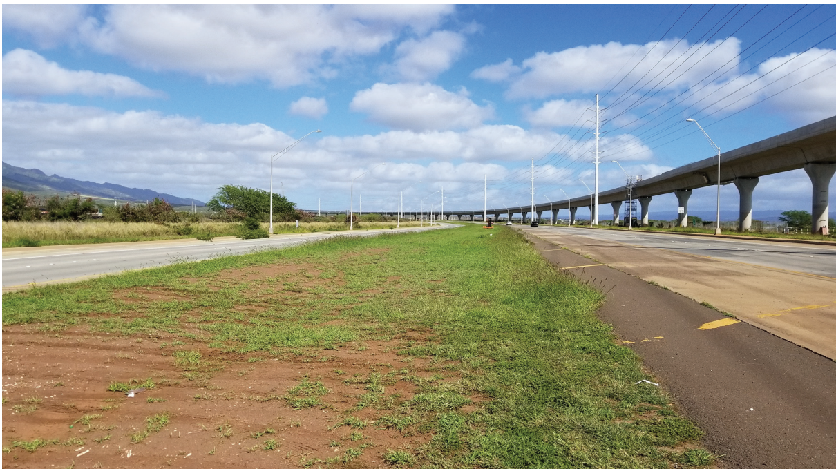
Fig. 1. Section view of a bioswale in practice along Kualakai Parkway road in Kapolei, Oahu, Hawaii.
