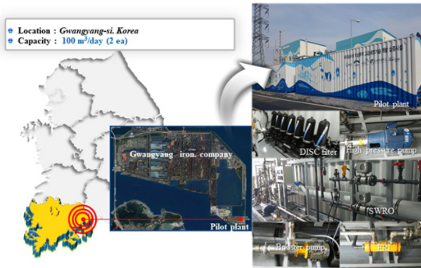
Fig. 1. Location of the SWRO desalination plant and picture of the pilot plant.
