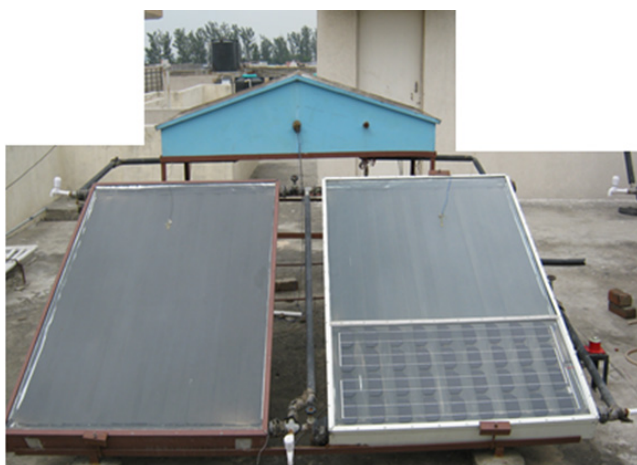
Fig. 3. Integrated flat plate collectors (FPCs) and modified double slope solar still.
