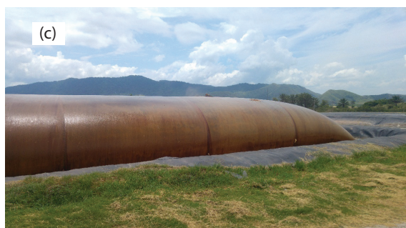
Fig. 2. (a) Sludge from evaporator; (b) sludge from lime treatment in a geobag and (c) details about geobag used for sludge dehydration.
