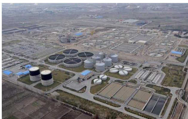
Fig. 1. Aerial view of Southern Tehran Wastewater treatment plant.
