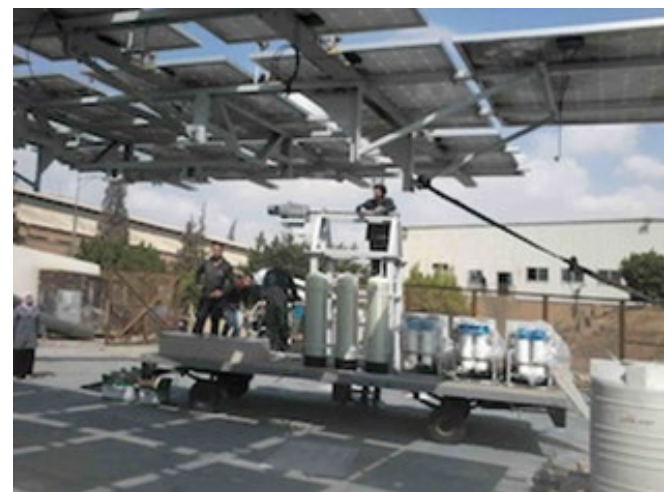
Factory testing of Shalateen unit
