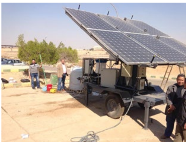
Factory testing of North coast unit
