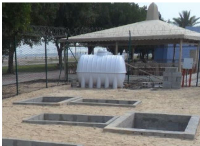
Fig. 2. Supply main tank and liner sections tested in the field.
