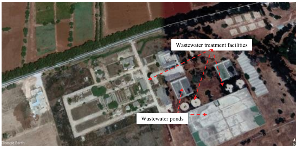
Fig. 1. Photograph shows the wastewater treatment plant in Al-Marj city, Libya.
