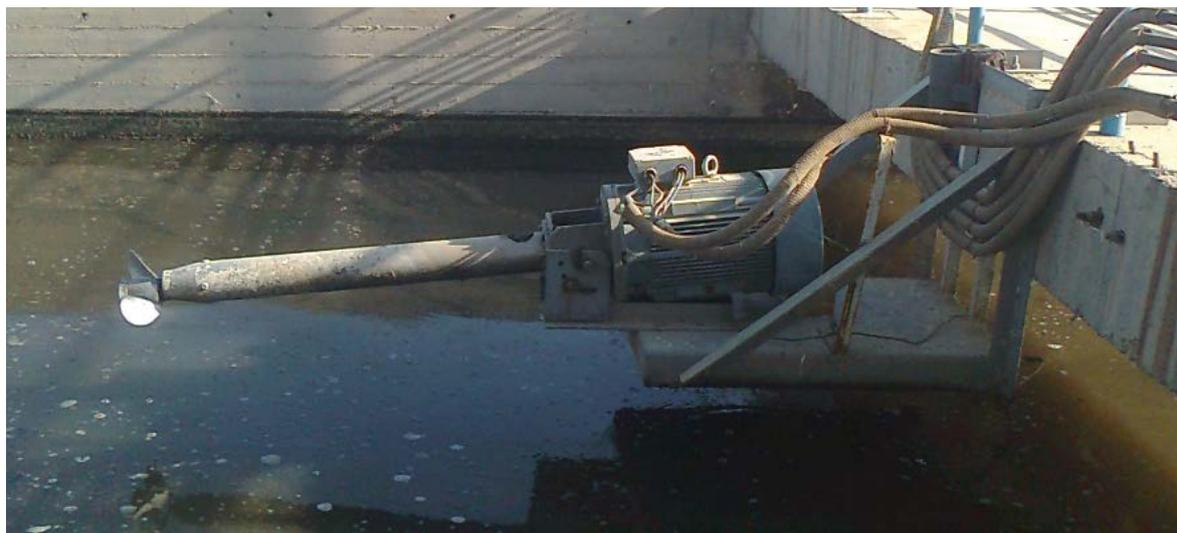
Fig. 2. Photo of a propeller-aspirator-pump used in Kermanshah's WWTP.
