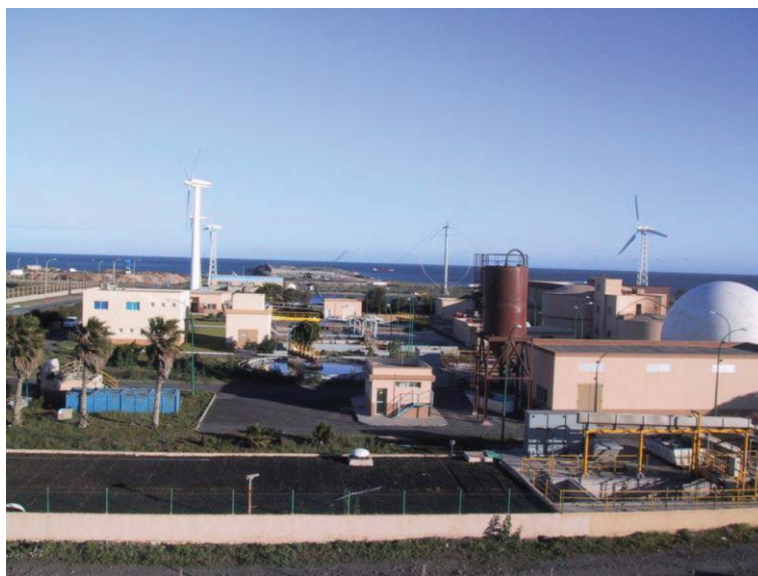
Fig. 4. View of the WWTP of the Southeast of Gran Canaria.
