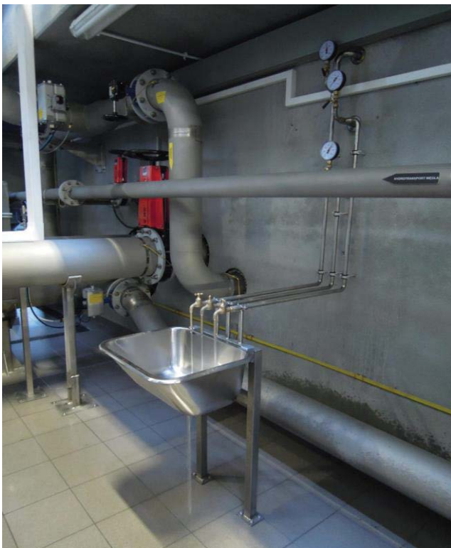
Fig. 3. Installation for collecting water from the filter bed cross-section.
