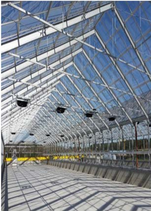
Fig. 1. Solar sludge dryer.
