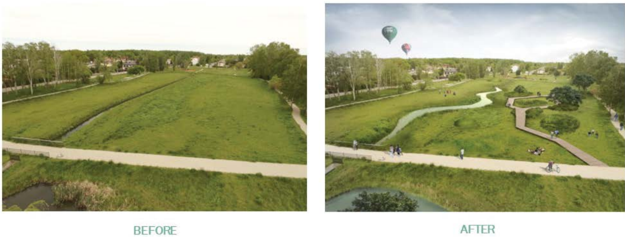
Fig. 12. Local recreation hub, Wasiaka Dry Reservoir area – Zone C. BEFORE: existing dry retention reservoir (occasional floodplain) and, Sokółówka River – heavily modified water body; AFTER – watercourse meandrization, dry reservoir bed diversified with mounds and depressions, hydrophyte planting, wooden deck – recreational and educational path. Source: Excerpt from final concept design, Studium – Workshop of Architecture.
