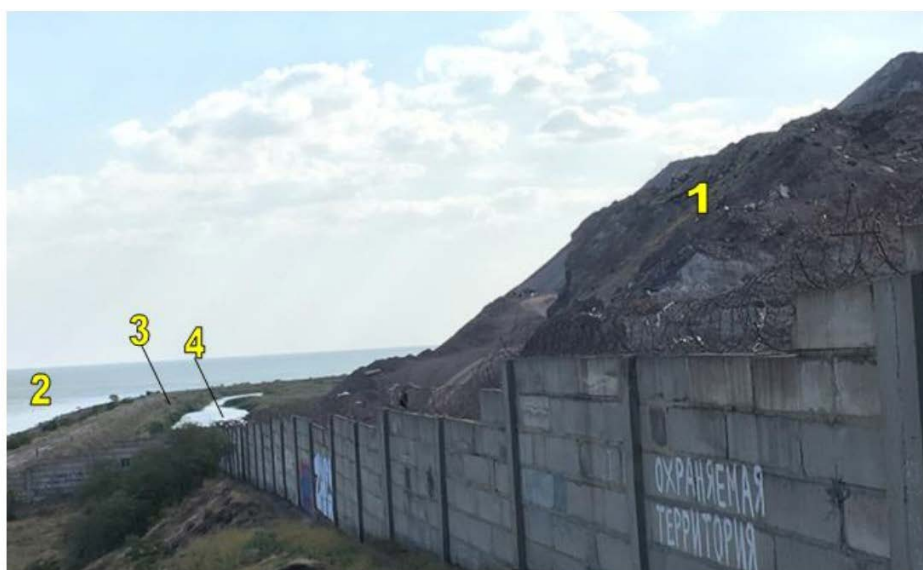
Fig. 1. Slag disposal of AZOVSTAL IRON & STEEL WORKS: 1 – slag disposal; 2 – the Sea of Azov; 3 – protective dam; 4 – slag infiltrate storage reservoir.
