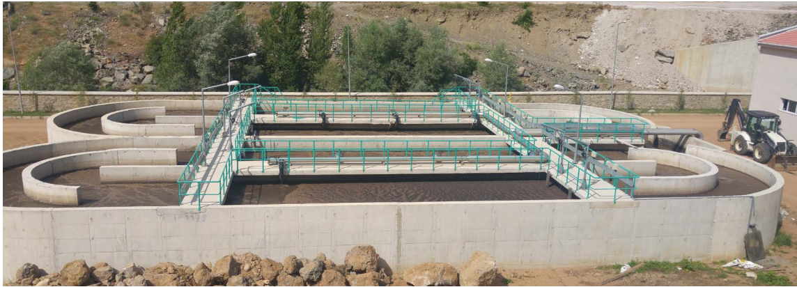
Fig. 1. The Gümüşhane oxidation ditches.
