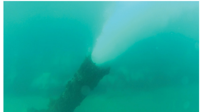
Fig. 1. Photo of the brine discharge diffuser of Fouka station.
