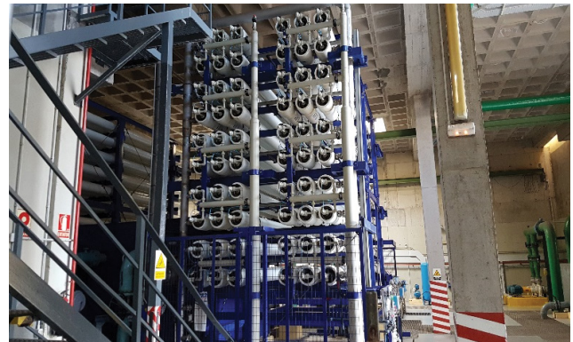
Fig. 1. Train with TFN membranes installed.
