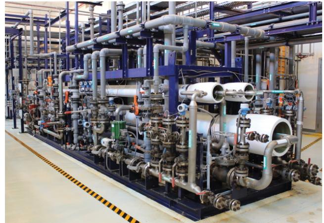
Fig. 6. RO section of the MEIC testing asset, used for the Red Seawater field trials.
