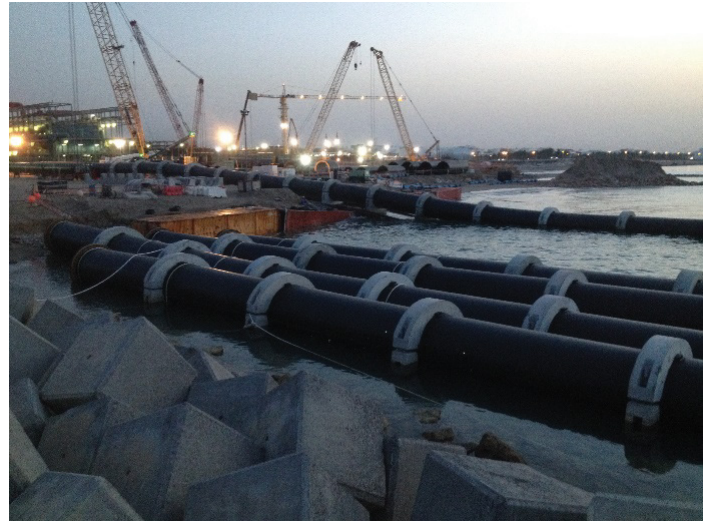
Fig. 10. Al Ghubrah desalination plant diffuser section and launching of the pipes.
