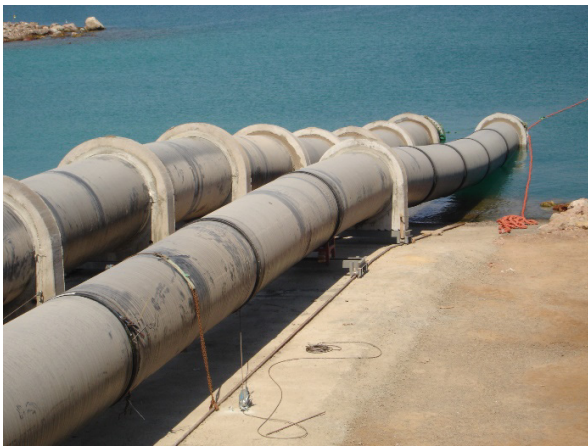
Fig. 8. Valdelentisco desalination plant launching of the pipes. The lower part of the riser can be seen in the right photo.
