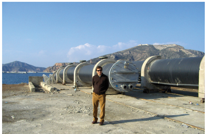
Fig. 8. Valdelentisco desalination plant launching of the pipes. The lower part of the riser can be seen in the right photo.
