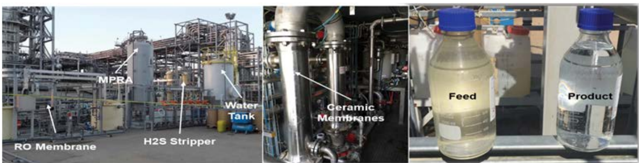
Fig. 8. Produced water desalination: membranes at field site.
