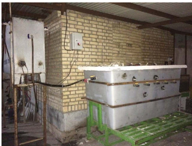
Fig. 2. The view of the API and AFR for the Kanyar dairy waste water treatment.
