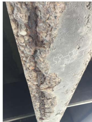
Fig. 2. Exposed T-beams.
