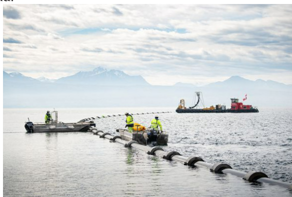
Fig. 1. floating HDPE Pipeline before sinking to the ground
