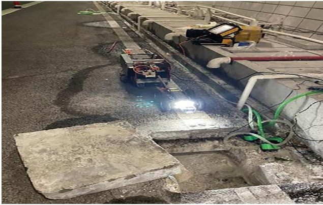
Fig. 10. Tunnel detection by pipeline crawling robot.
